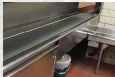
COMPLETED BELT TO DROP-OFF
